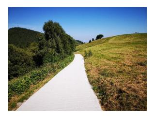
The ground is cemented, with small grooves that allow rainwater to run off.
