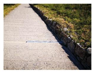
On the right half of the road uphill, we pass some gratings, which allow us to cross some grooves for rainwater to run off.
