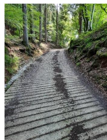
The bottom is now cemented with joints for the water to flow, the slope is fair and constant.
